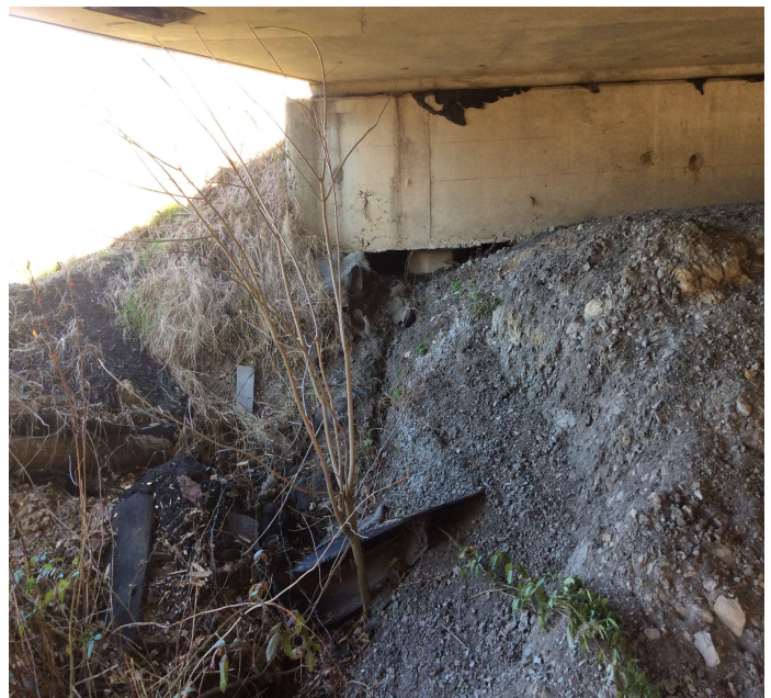
PHOTO 2 Description Erosion under bent 7 cap left side
