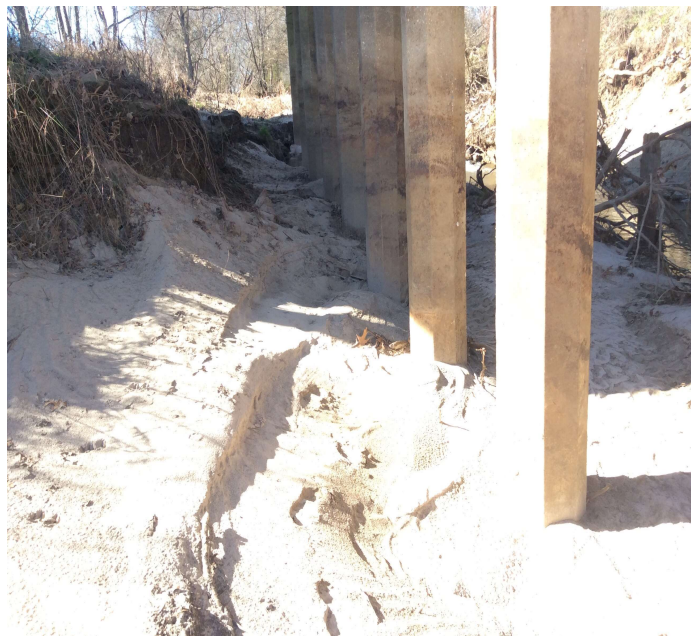
PHOTO 1 Description Erosion bent 4
