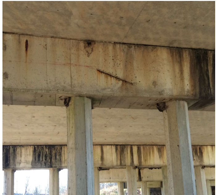
PHOTO 6 Description Bent 5 cap west face rebar exposed
