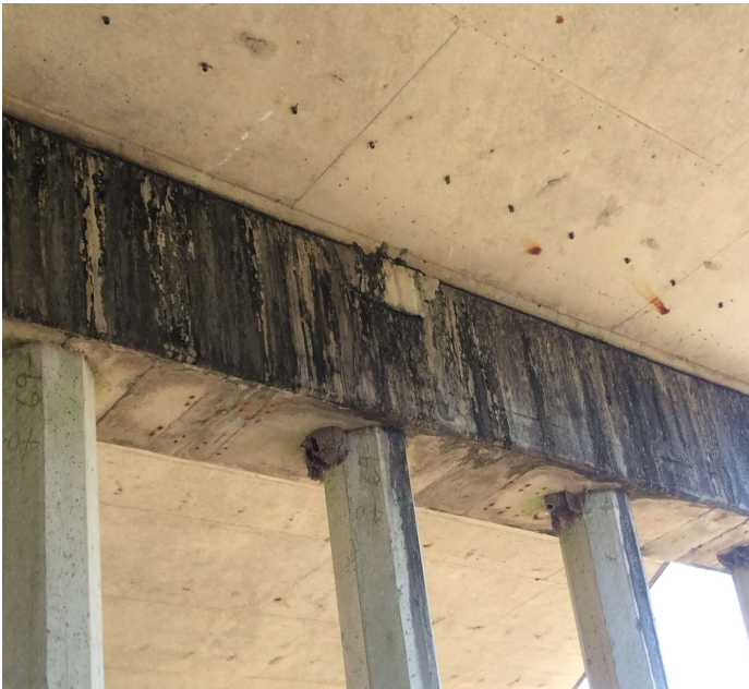
PHOTO 4 Description Bent 4 west face delam
