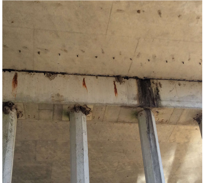
PHOTO 5 Description Bent 5 west face spalls
